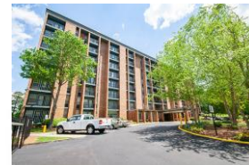
East Lake High-rise above; 149 units.
